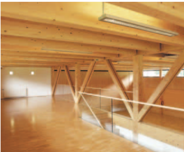
Use of KLH rib elements at an event hall
