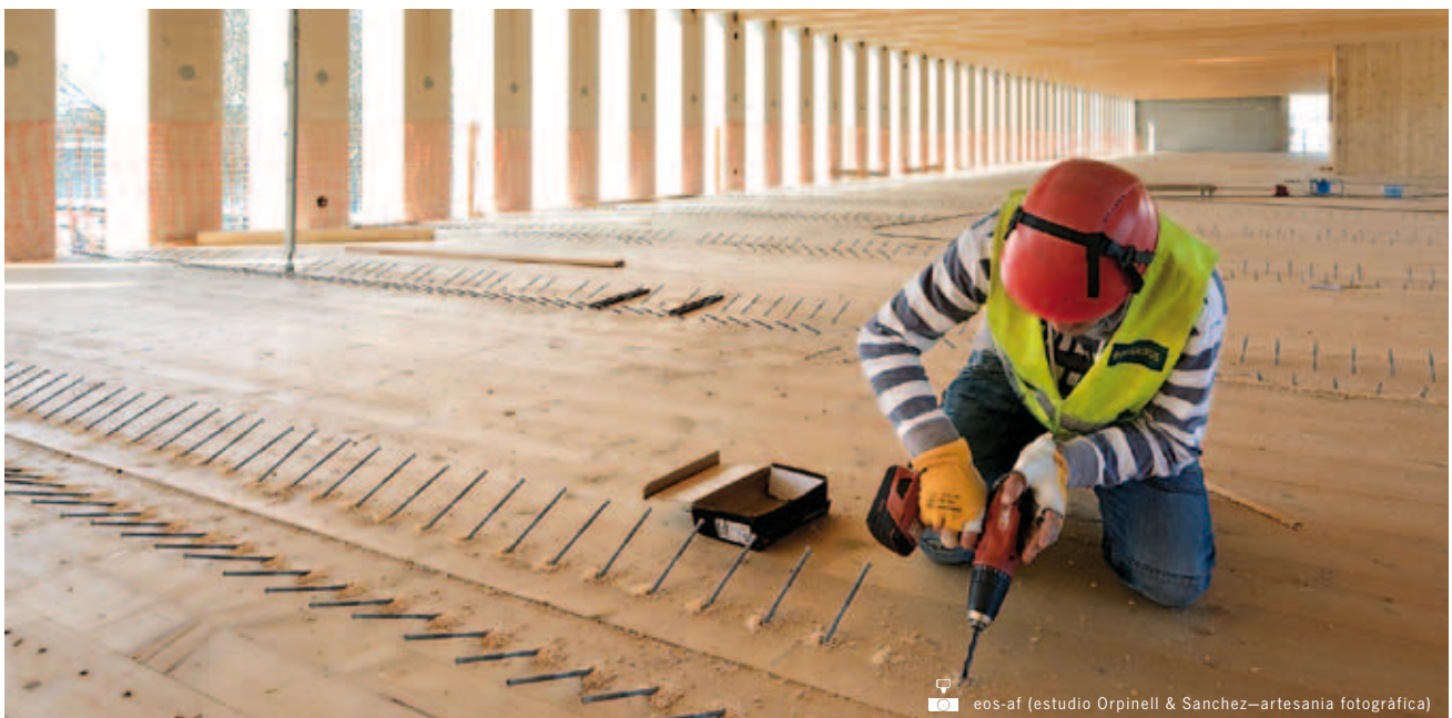
Making of transverse connections
