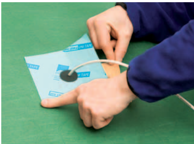
Fig. 10: If the penetrations cannot be avoided, suitable and approved systems should be used for sealing. A quick and permanently tight mounting will justify the additional costs [with the kind support of the company pro clima 2011].
